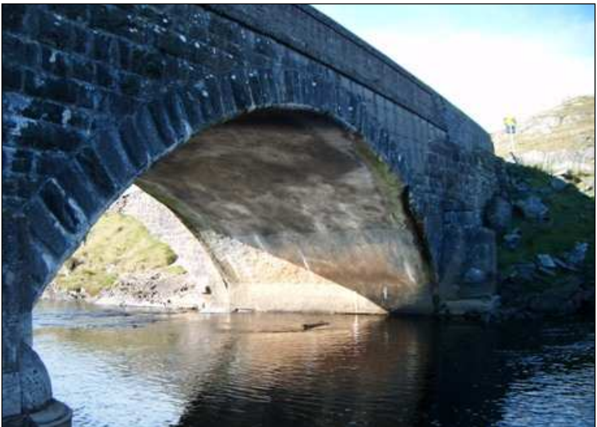
Plate 12: Canal Bridge GC-N59-026-00 at Chainage 237120
