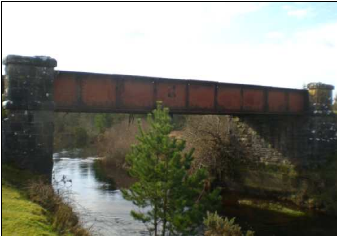
Image 2.4 Oughterard River Bridge currently in place
