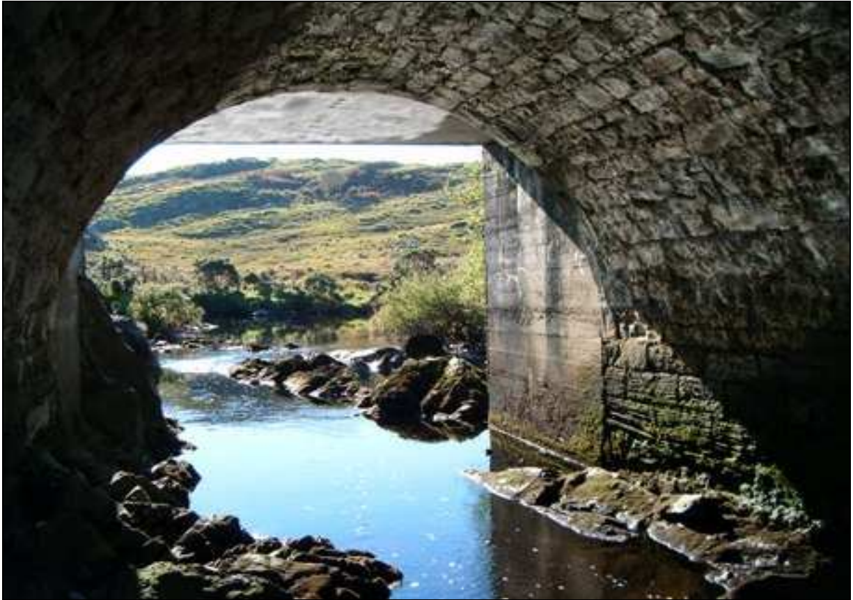
Plate 11: View beneath Glencoaghan Bridge GC-N59-025-00 at Chainage 236530
