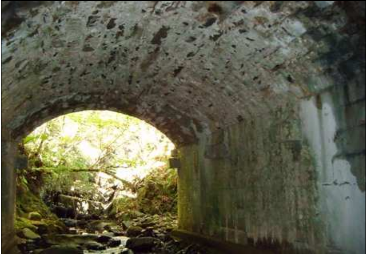
Plate 9: View beneath Emlaghdauroe Bridge GC-N59-023-00 at Chainage 232380
