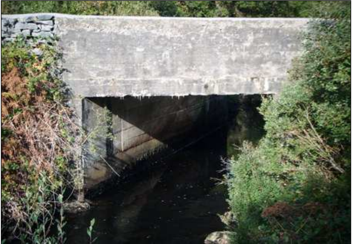
Plate 17: Bridge GC-N59-030-00 at Chainage 246440
