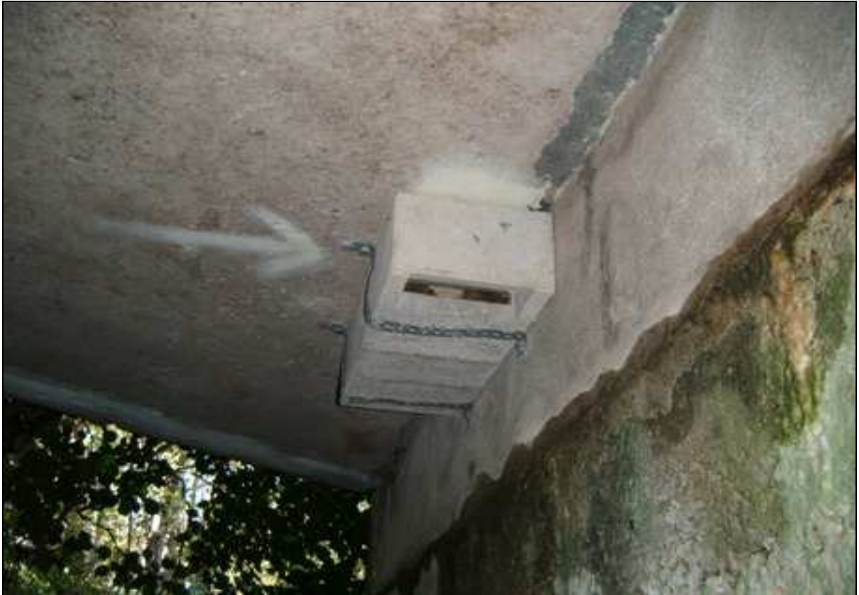
Plate 5: One of two bat tubes installed on bridge GC-N59-022-00 at Chainage 231200
