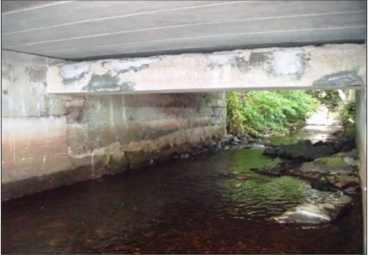
Plate 19: View beneath Lurgan Bridge GC-N59-036-00 at Chainage 254820
