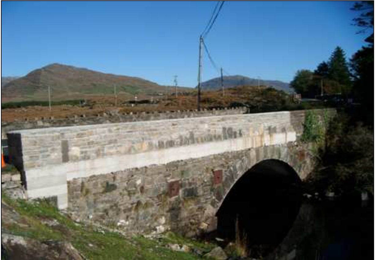
Plate 13: Weir Bridge GC-N59-027-00 at Chainage 241070
