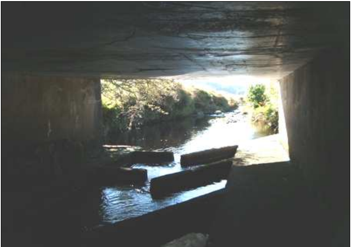
Plate 10: View beneath Lettery Bridge GC-N59-024-00 at Chainage 234420
