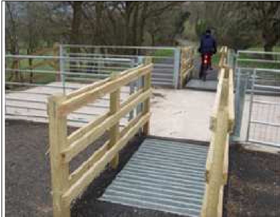
Image 2.2 Example of Greenway Section with Cattle Stops
