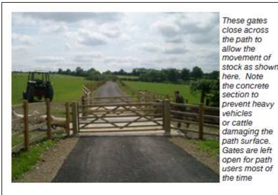
Image 2.3 Example of Greenway Section with Cattle Stops
