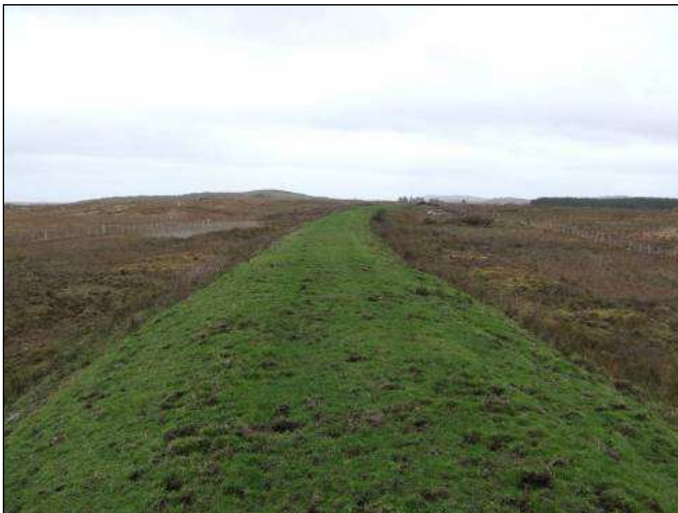
Image 3.1 An example of the proposed route and former railway within townland of Emlaghmore, facing west, with improved topsoil raised above the surrounding bog.
