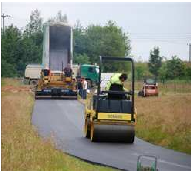
Image 2.1 Example of a similar final surface being laid
