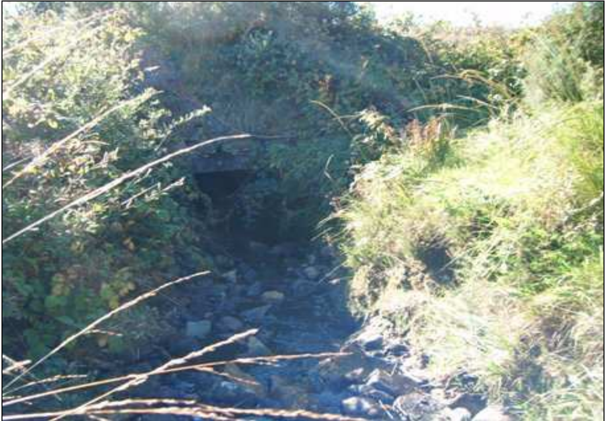
Plate 3: Low bridge GC-N59-021-00 at Chainage 230750
