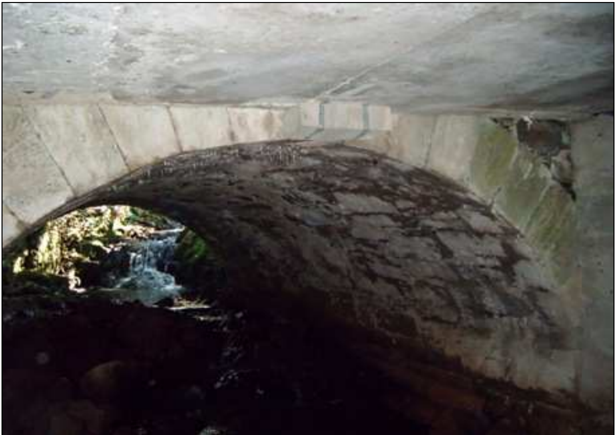
Plate 6: View beneath bridge GC-N59-022-00 at Chainage 231200 showing second bat tube
