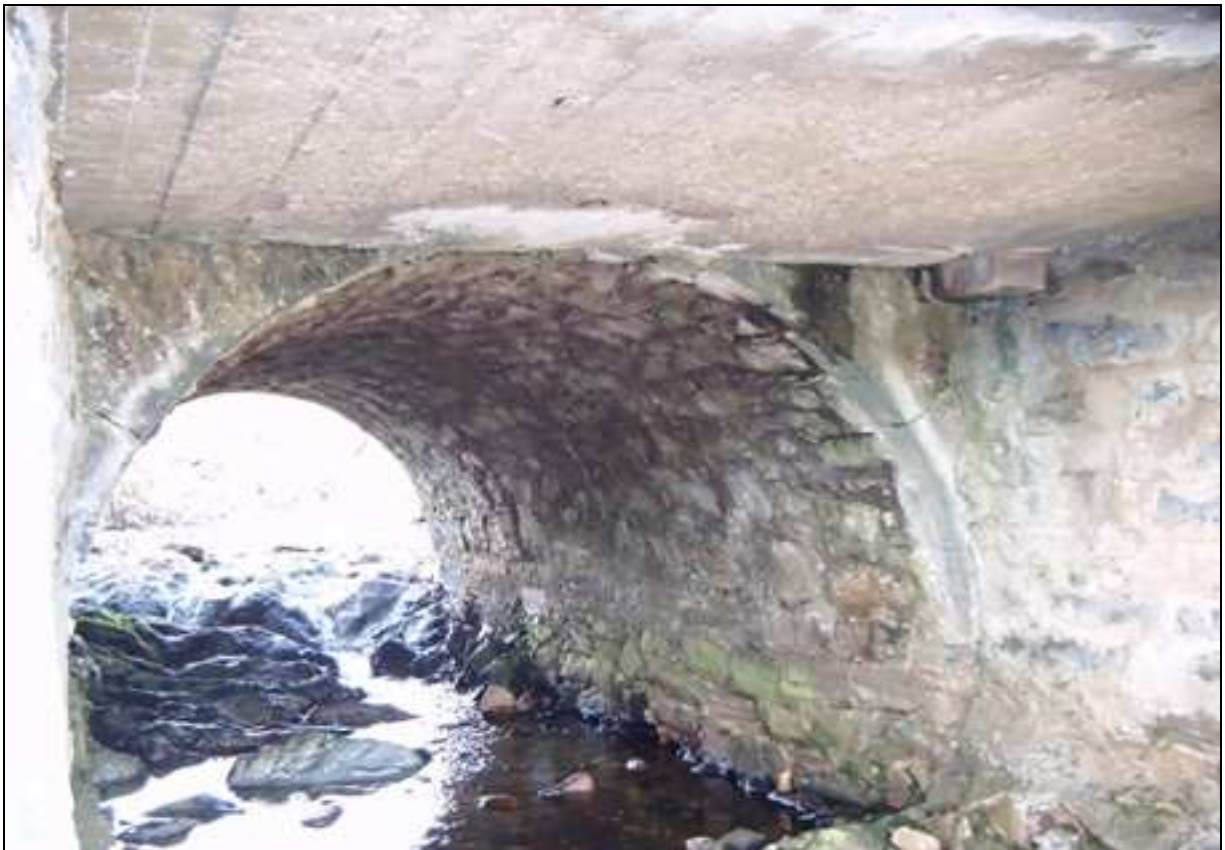
Plate 18: View beneath Bunsconnive Bridge GC-N59-035-00 at Chainage 251770 - bat tube at right
