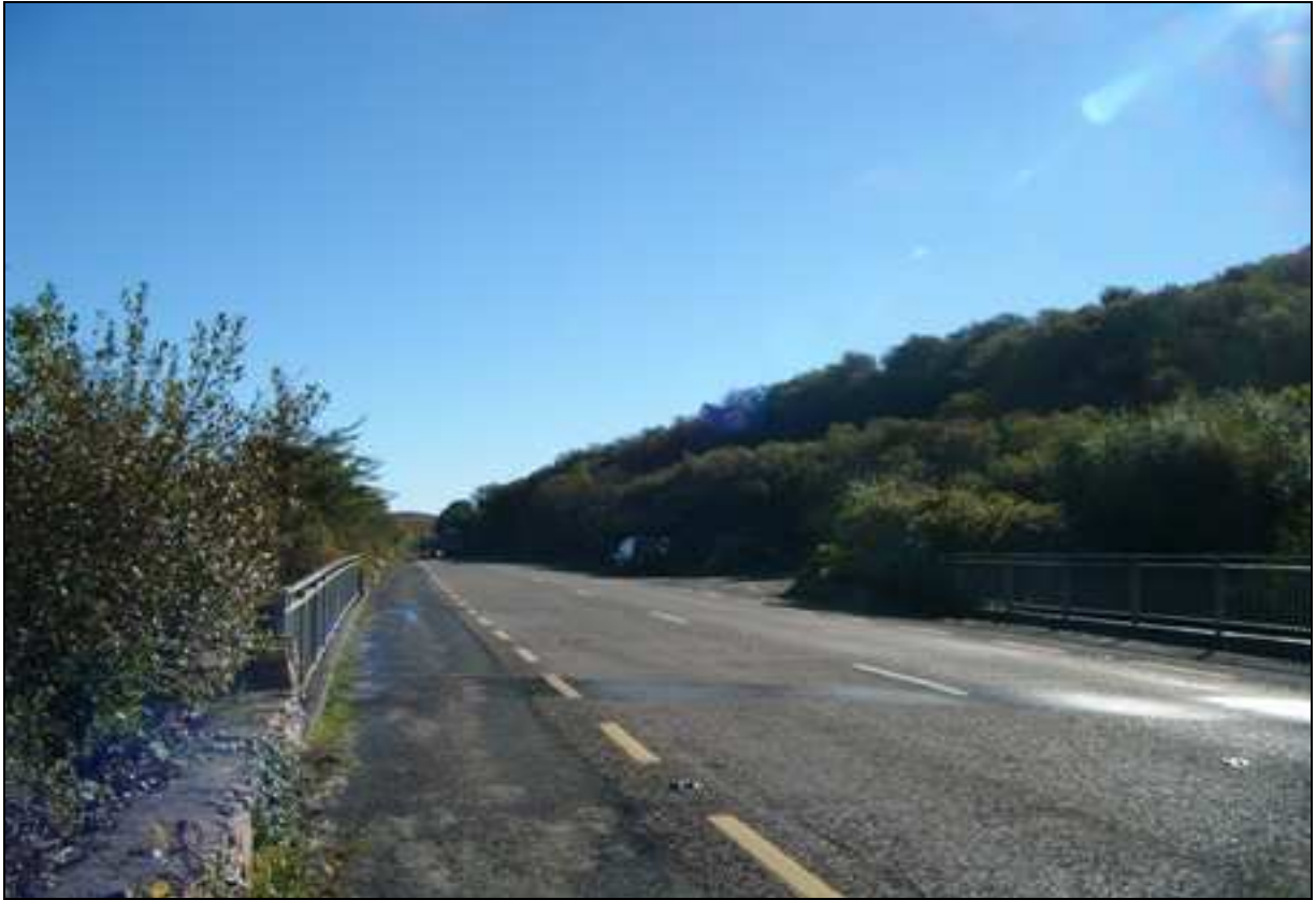
Plate 1: View east along existing N59 at Chainage 223650 over bridge GC-N59-020-00
