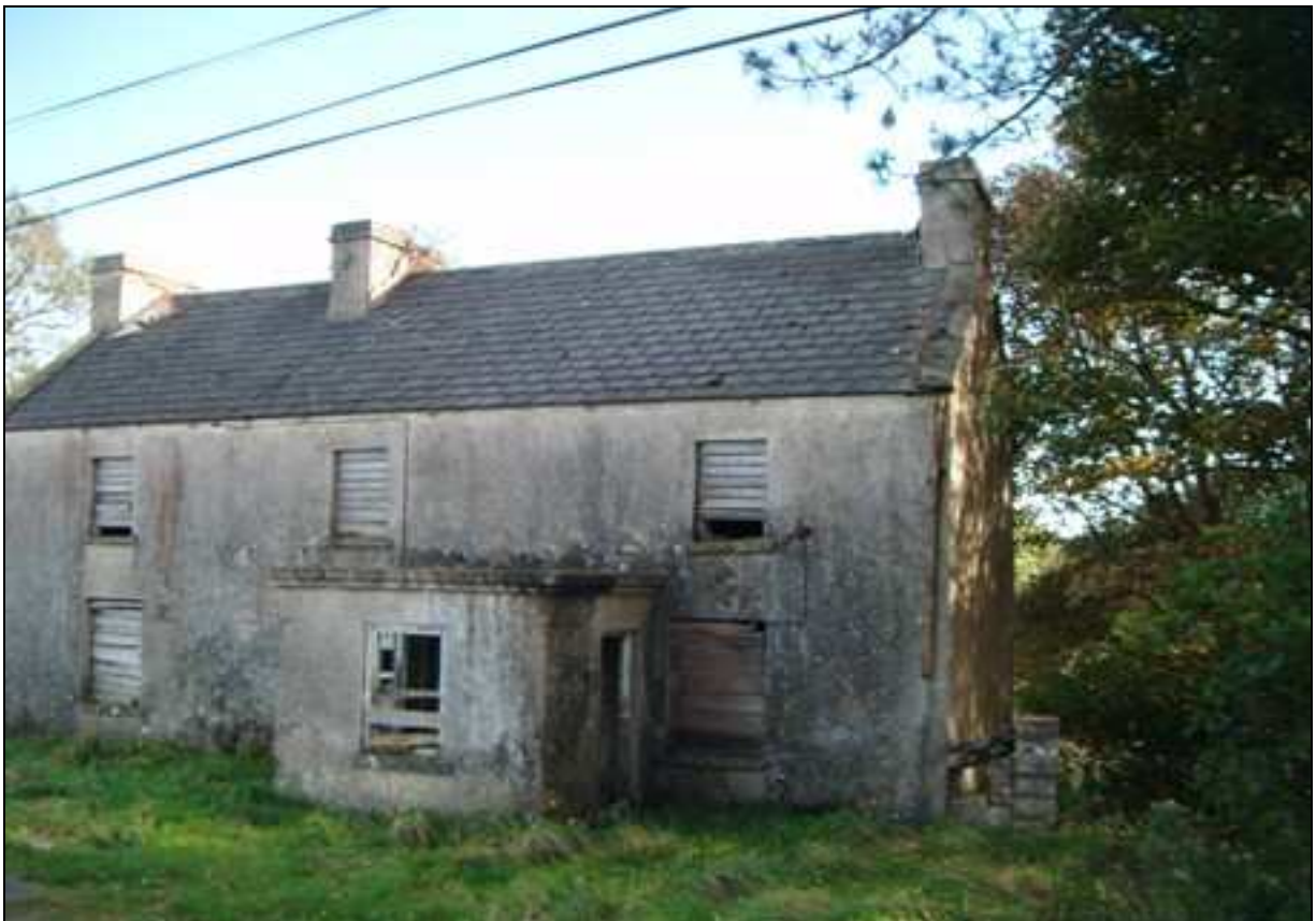
Plate 16: Derelict two-storey dwelling immediately south of existing road at Chainage 244740
