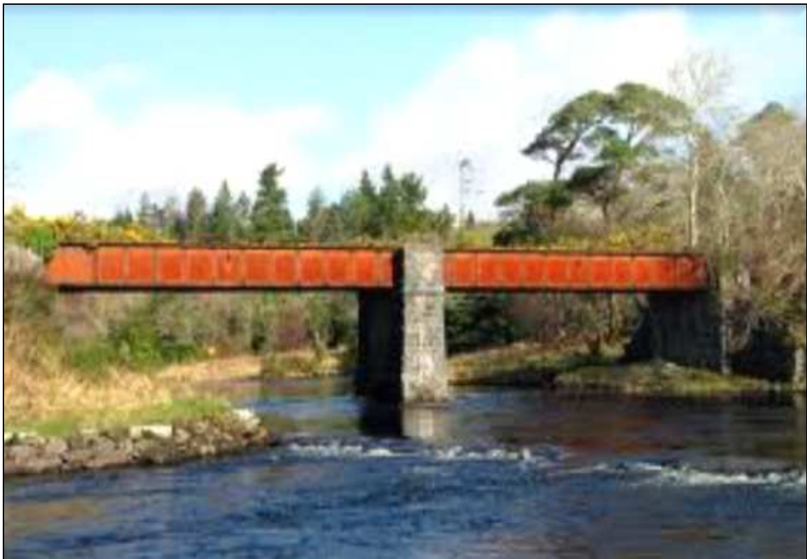
Image 2.6 Cloonbeg River Bridge currently in place
